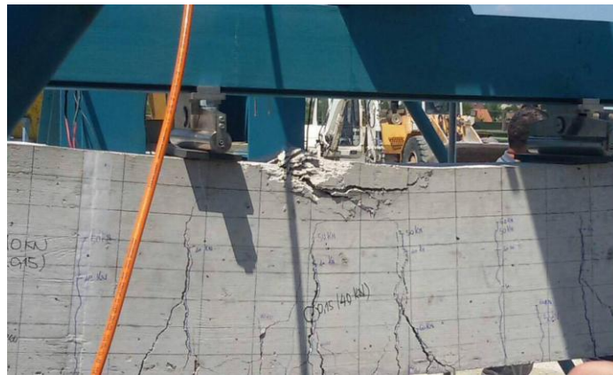
Figure 15. Crack distribution and failure locations at the ultimate load stage
