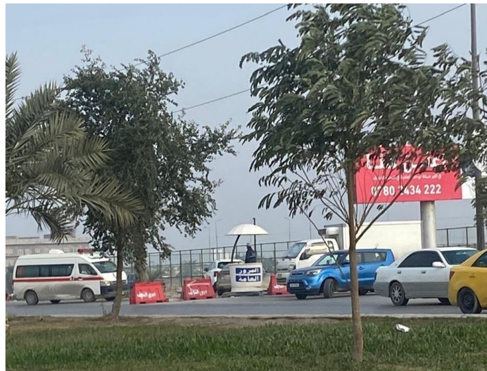
Figure 9. Unacceptable U-turns radius of the original design, using plastic barriers to reduce the significant influence
