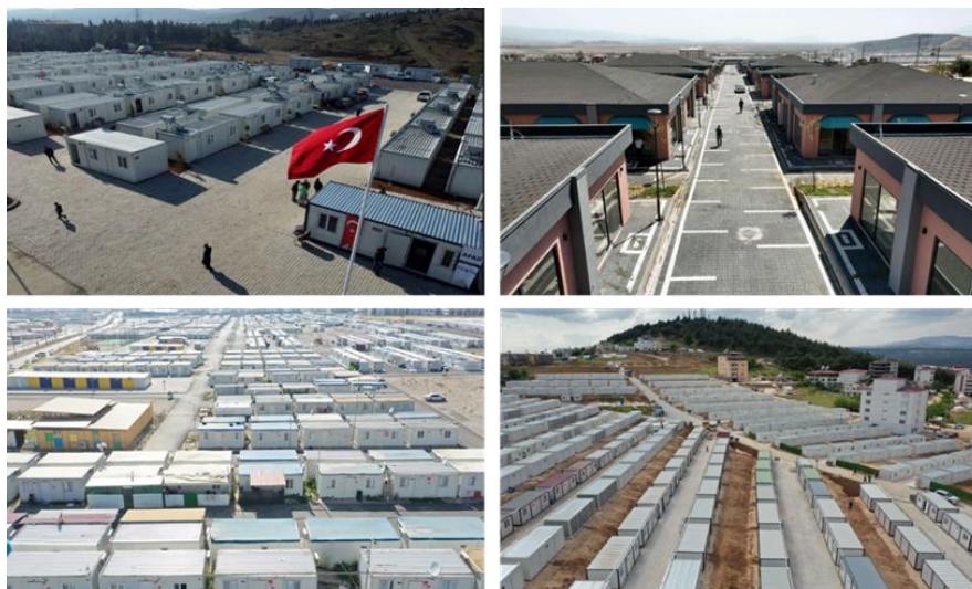
Figure 11. Representative container-settlement layouts in Gaziantep and Kahramanmaraş [15]
