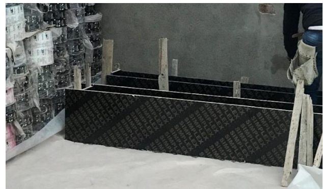
(b) Plywood Form of the Beams
