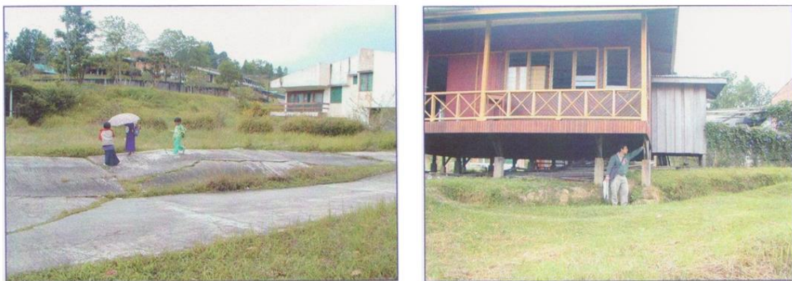
Figure 4. Ground deformation at SMK Kundasang caused by progressive soil movement [19]
