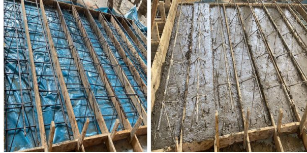
Figure 6. Reinforcement and casting of slabs
