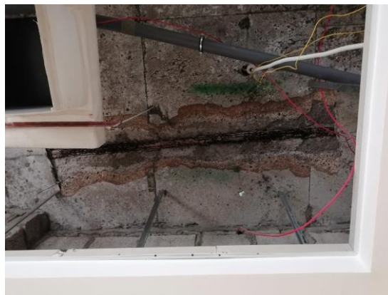
Figure 8. Exposed and corroded PT strands at roof slab soffit
