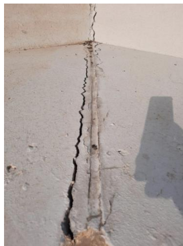
Figure 12. Damaged expansion joint
