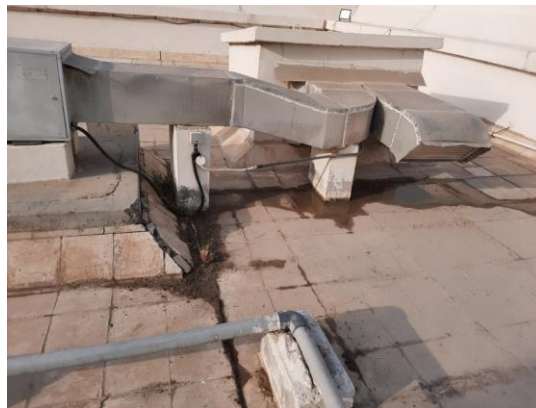
Figure 10. Leakage in the roof slab
