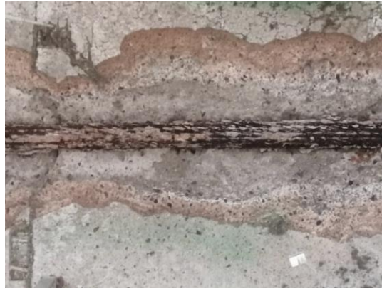
Figure 9. Delamination and spalling of exposed corroded rebar in the roof beam
