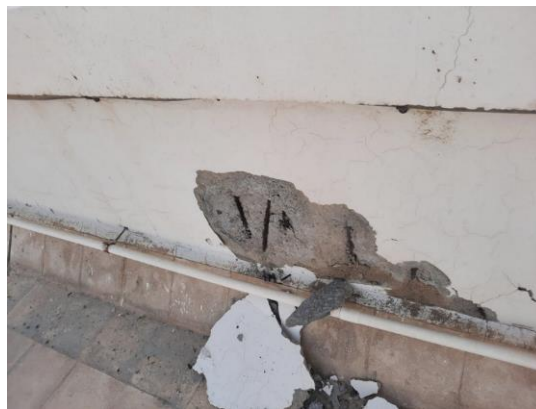
Figure 11. Delamination/spalling of the concrete in the parapet
