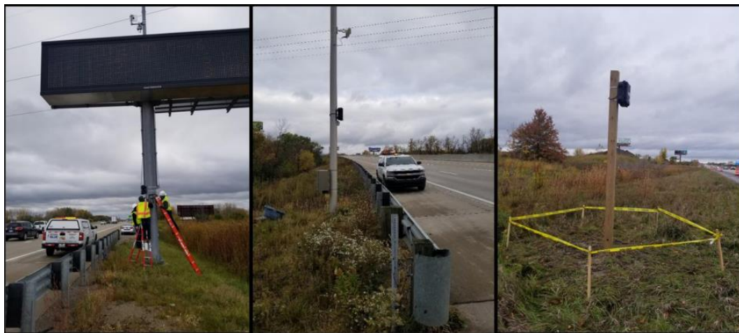
Figure 3. Examples of sensor mounting mechanisms
