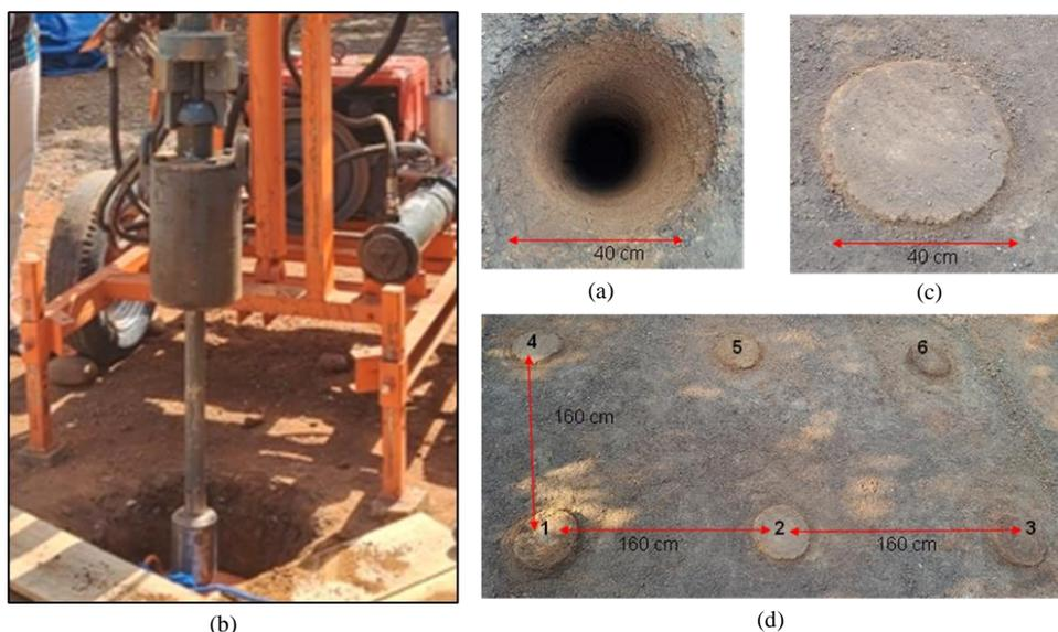
**Figure 5. The compaction process of column**
