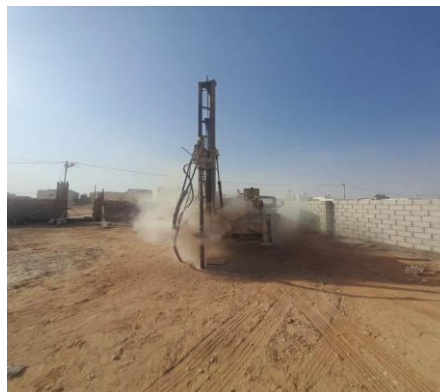
Figure 9. Drilling and sampling (Al-Mafraq)
