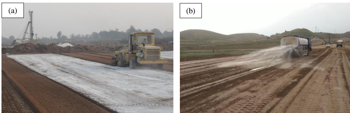
Figure 6. (a) Soil stabilizing mixer; (b) Sprinkling truck
