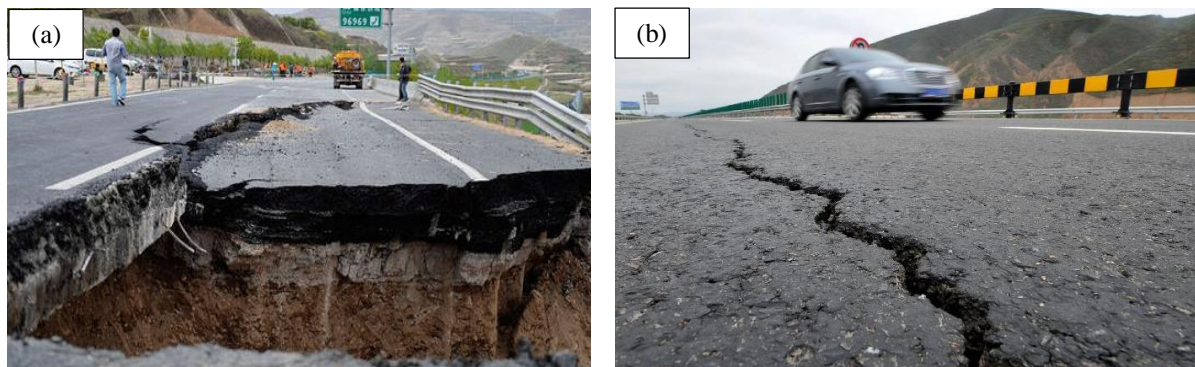
Figure 2. Highway hazards in Loess Plateau area. (a) Embankment hazards of Tianding highway; (b) Pavement hazards of Yanyan highway
