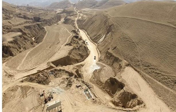
Figure 5. In situ test site (Wuding highway)
