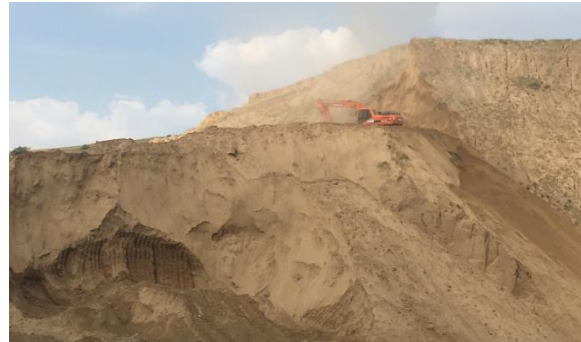
Figure 3. Borrow pit 1# (located at Wuding highway)
