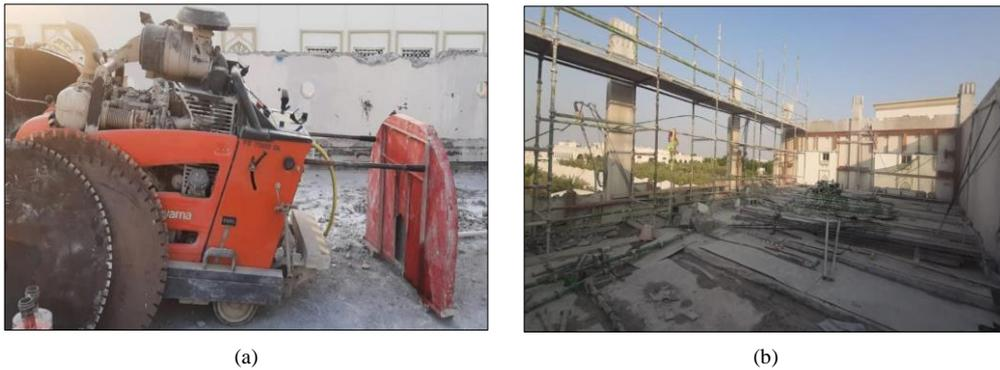
Figure 11. (a) Concrete cutting to remove significantly deteriorated slab; (b) Removed slab
