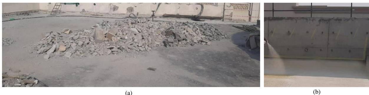
Figure 14. (a) Old waterproofing removal, (b) New waterproofing
