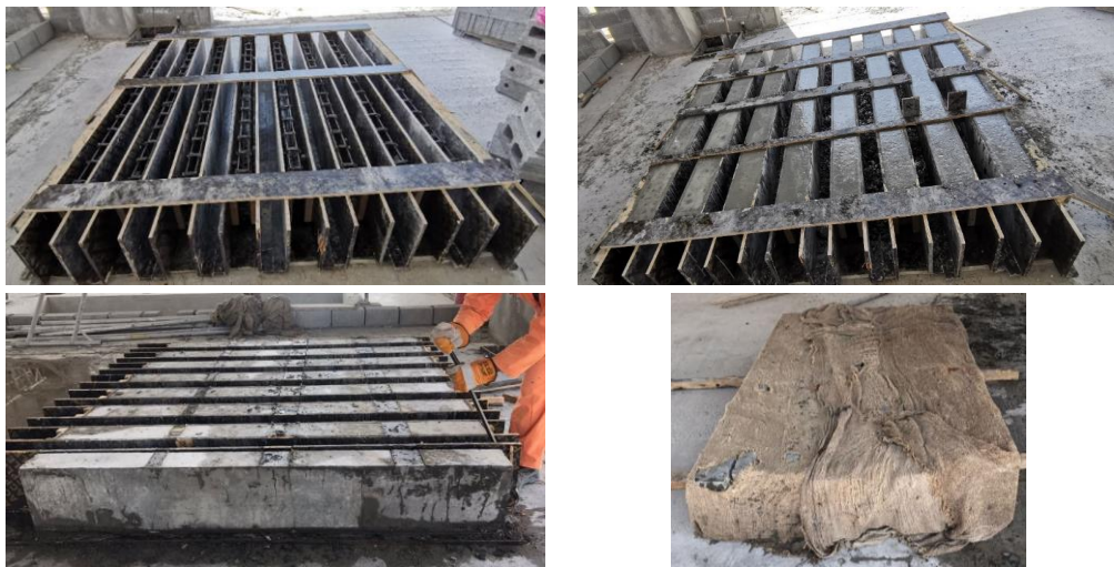
Figure 4. Casting of concrete beams
