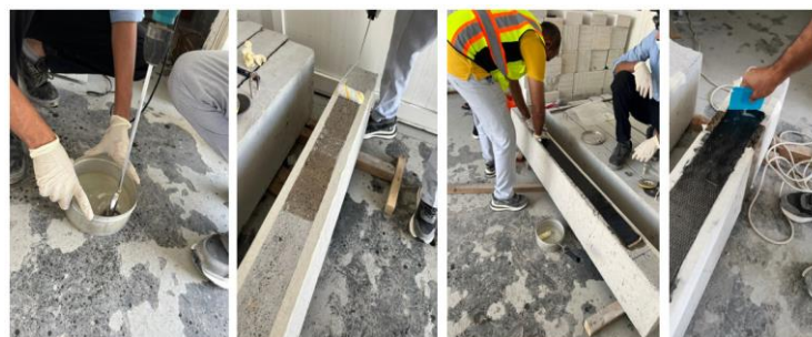
Figure 5. Externally Bonding CFRP to concrete Substrate
