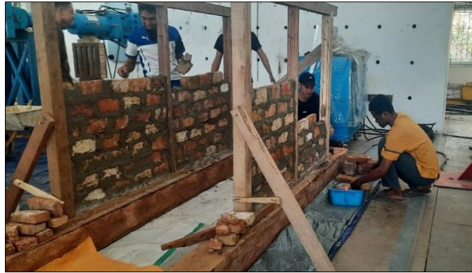
Figure 8. Process of installing a brick wall
