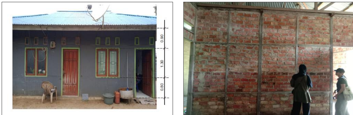
Figure 3. (a) A pattern of windows and doors frame that often appears in Kancingan house, (b) Timber frame pattern on wall in Kancingan house
