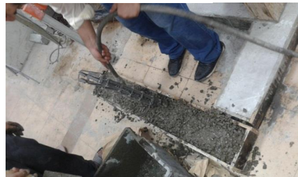
Step 2: Casting of the column
