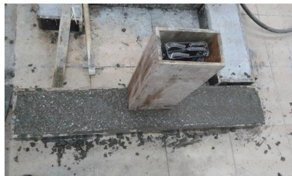
Step 3: Fixation and Casting of the beam
