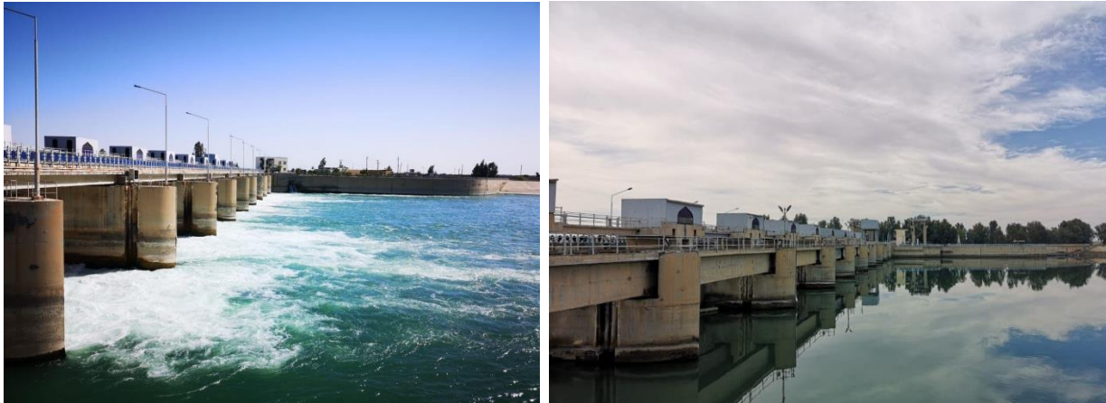
Figure 7. General view of Fallujah barrage from the upstream side (Photos taken on 15/5/2021)
