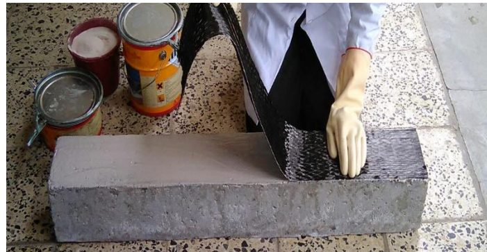
Figure 3. Strengthening beam with carbon fibers
